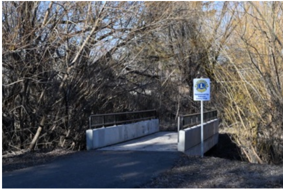
Yakima Lions Helped Build Bridge in Randall Park. Recently installed sign.
